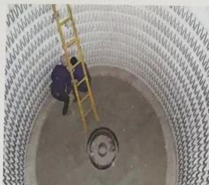
电加热炉 Electric heating furnace
