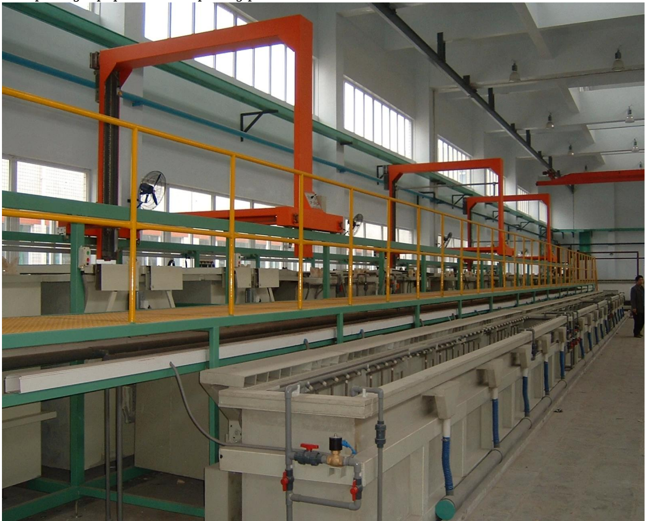
Zinc plating equipment . zinc plating plant.
