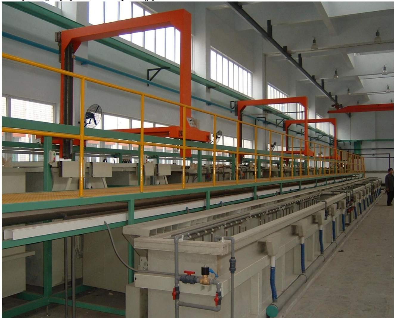
Zinc plating equipment . zinc plating plant.
