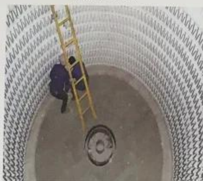
电加热炉 Electric heating furnace
