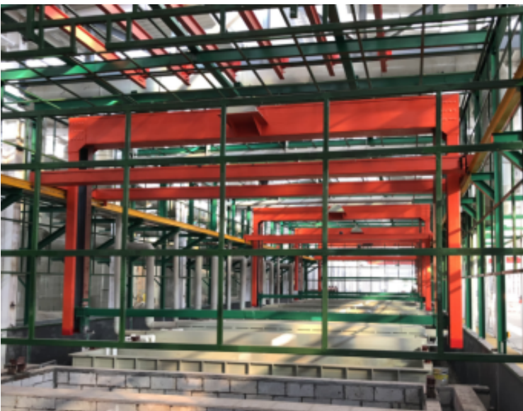
Fully auto acid washing crane
