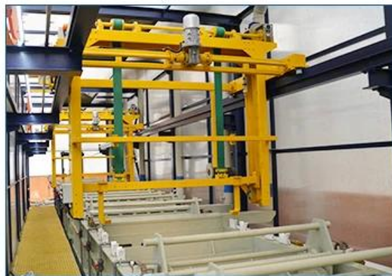
Zinc barrel plating line
