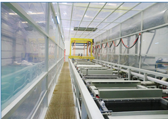
Phosphorization production line
